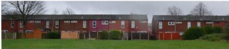
01. PHOTO OF EXISTING TERRACED HOUSES ON THE UPLANDS
